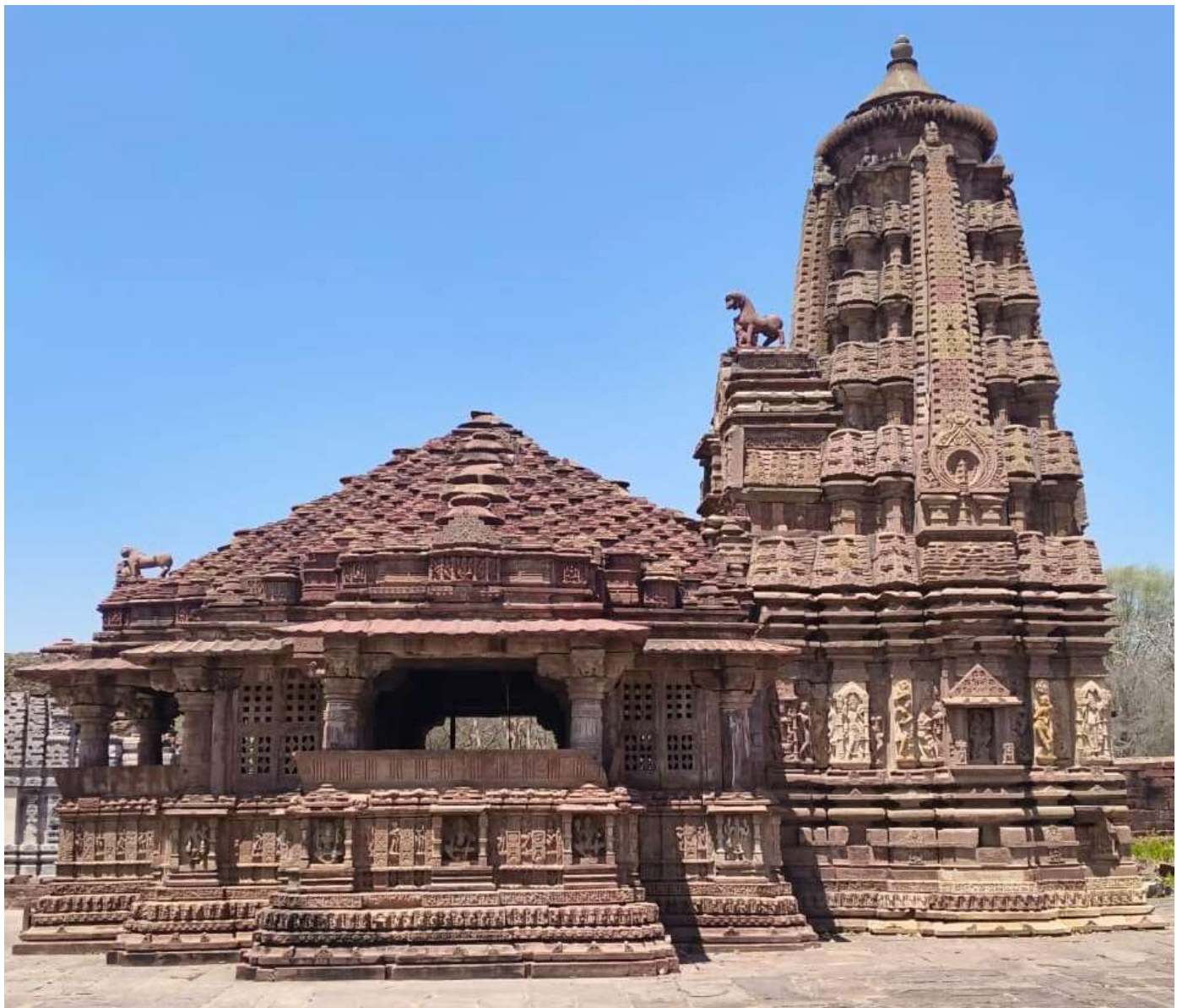
Fig. No. 04: North sided view of the Mahanal Temple, Menal, Chittorgarh.
