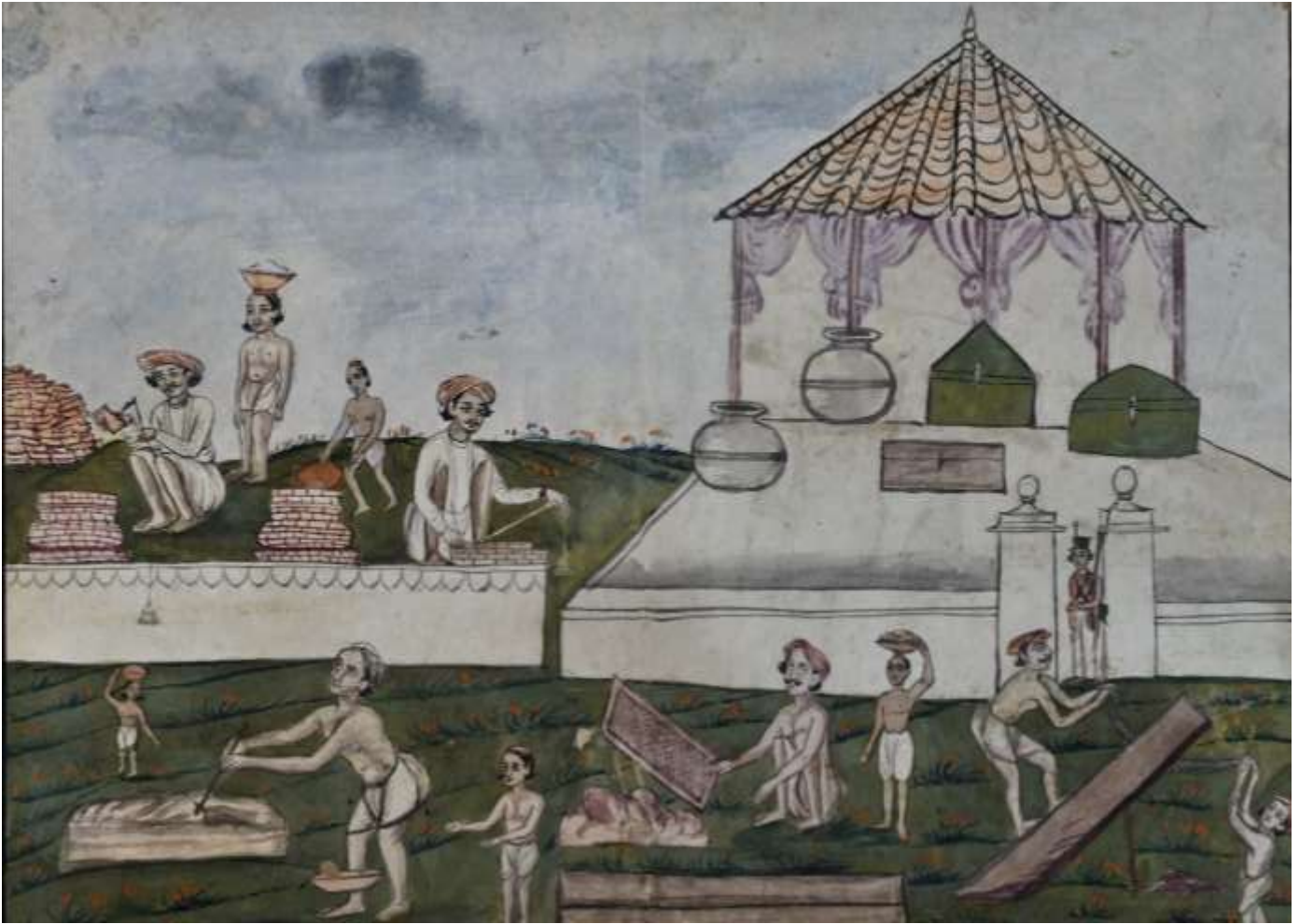
Fig no. 108: Scene of building construction.
