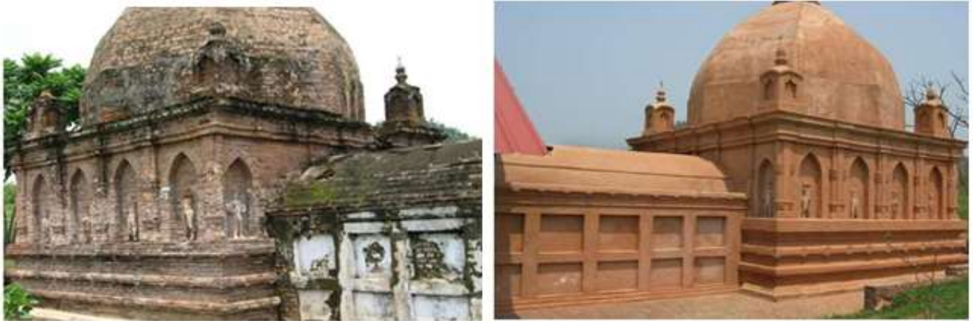
Figure 15: Kameswar temple before and after plastering of the main temple Source: (IAR 2009-2010: 279)
