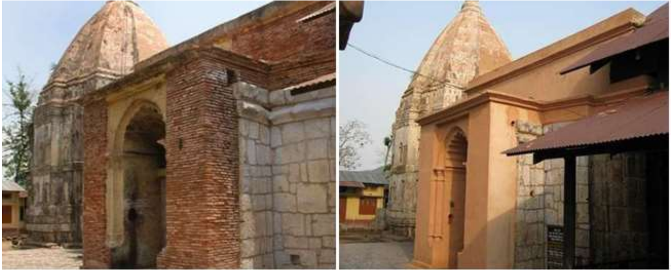
Figure 14: Hayagriva Madhava temple before and after plastering of the main temple Source: (IAR 2009-2010: 278)
