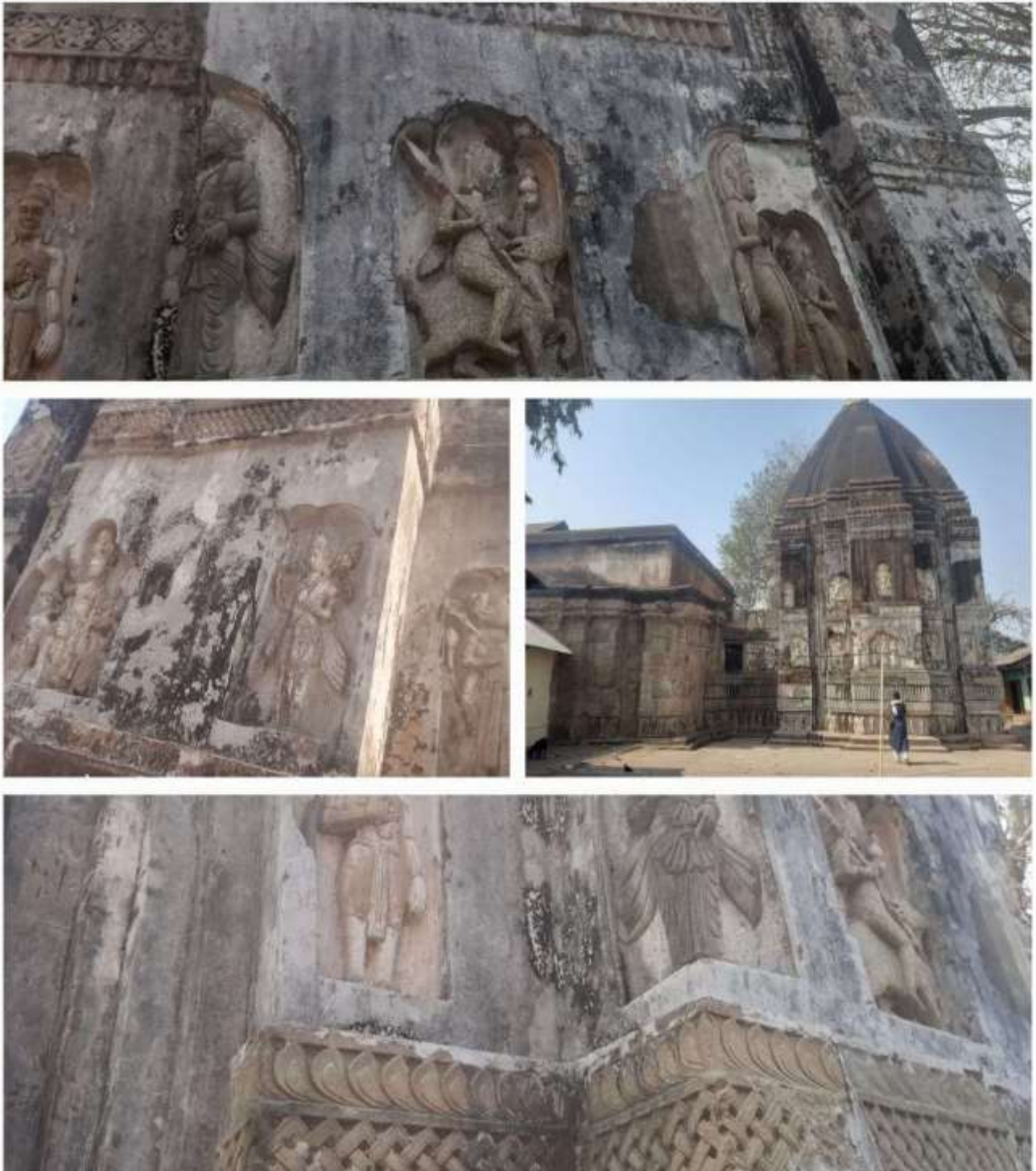
Figure 4: Sculptures on the exterior wall of the temple
