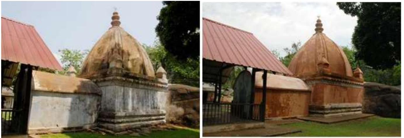
Figure 16: Ganesh temple before and after pastering of the main temple Source: (IAR 2009-10: 281)
