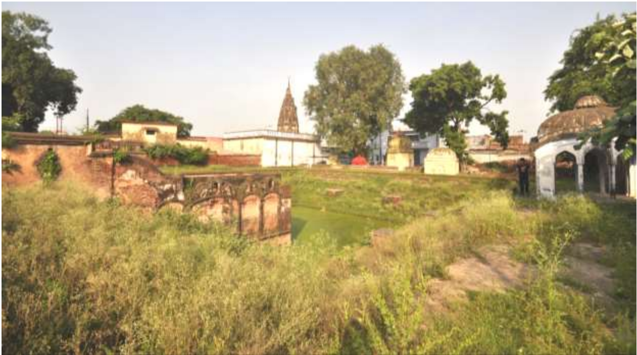
Fig. 25: Masonry Tank, Lala Moolchand Haveli
