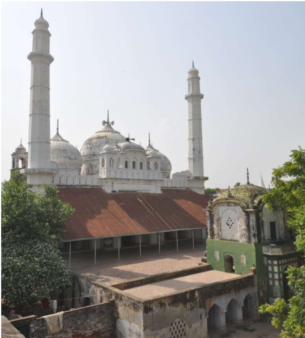
Fig. 58: General View of Jama Masjid
