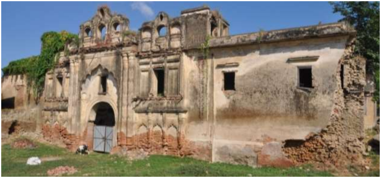
Fig. 96: Front façade of Imambara
