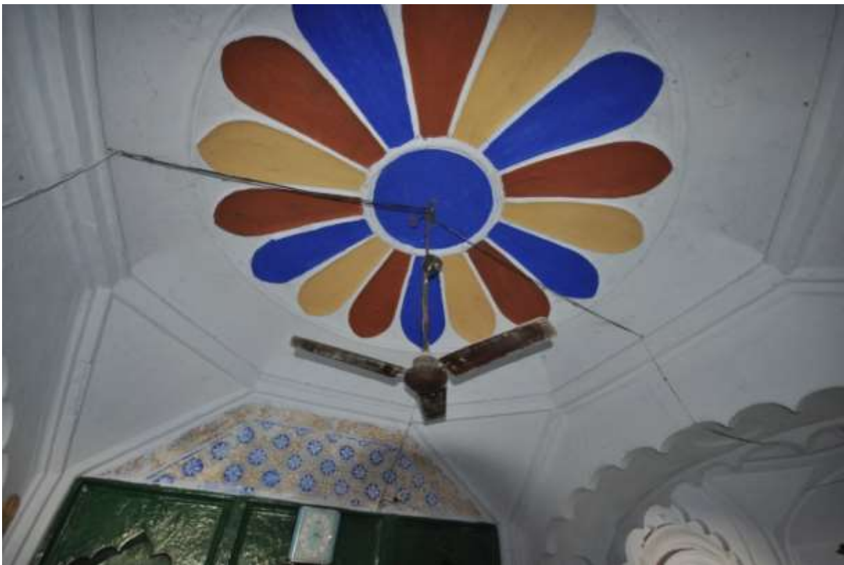
Fig. 87: Roof, Ghassoowali Masjid
