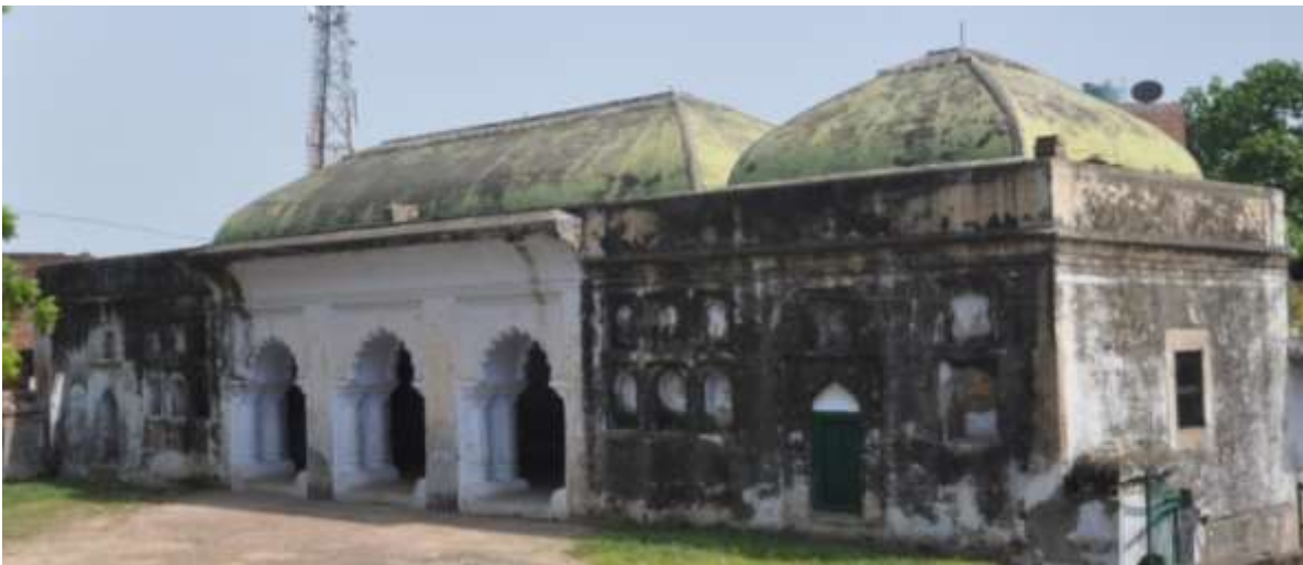
Fig. 57: Structure in South-east corner of the Complex
