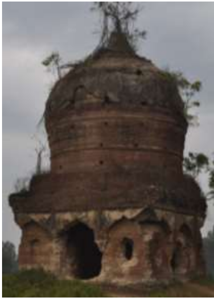
Fig. 230: General view of Aulia Bibi ka Math
