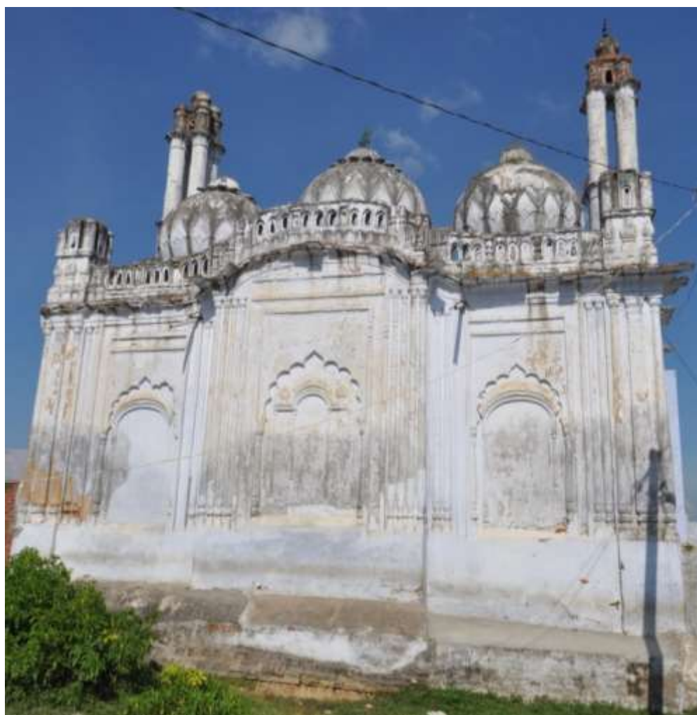
Fig. 85: Rear Façade, Ghassoowali Masjid
