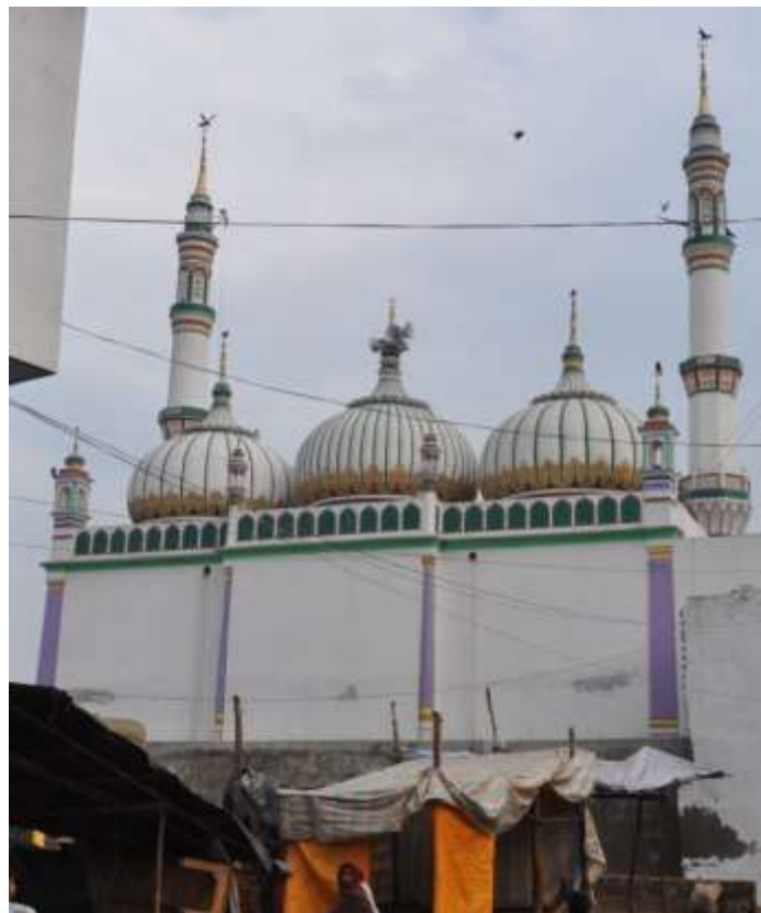
Fig. 245: Rear façade of Chhotii masjid
