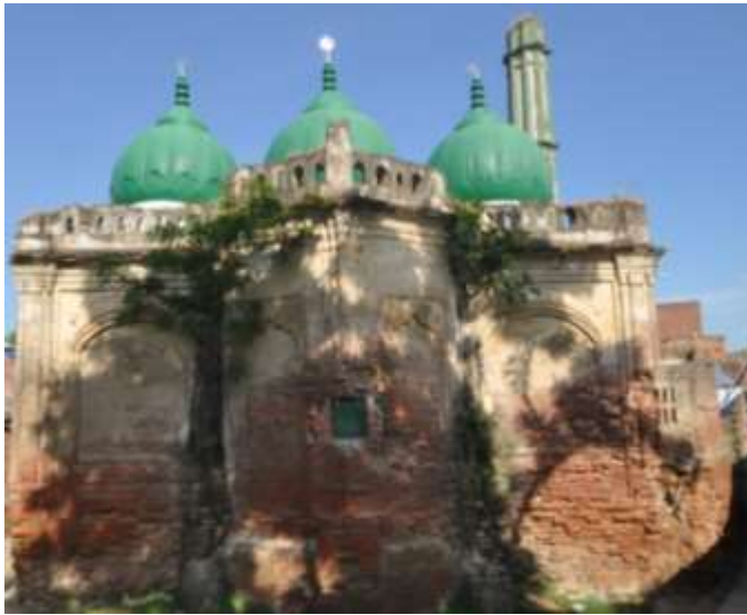
Fig. 101: Rear Façade of Takiya wali Masjid
