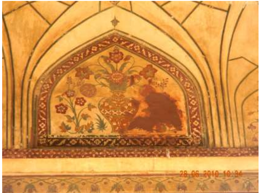
Fig. 12- Another View of Ceiling of Corner Pavilion, Salabat Khan
