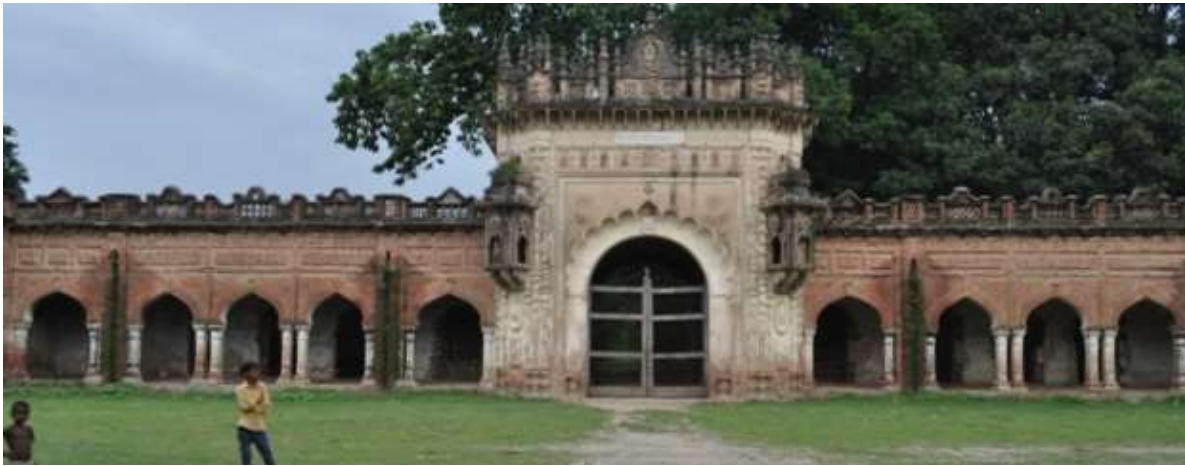
Fig. 78: Front gate, Ranibagh
