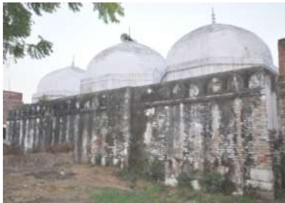
Fig. 284: Rear façade of Jama masjid
