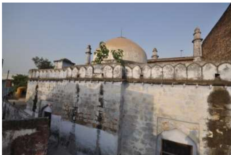
Fig. 66: Rear Façade, Kankar Wali Masjid
