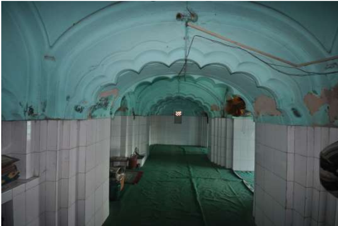
Fig. 308: Interior of Bari masjid
