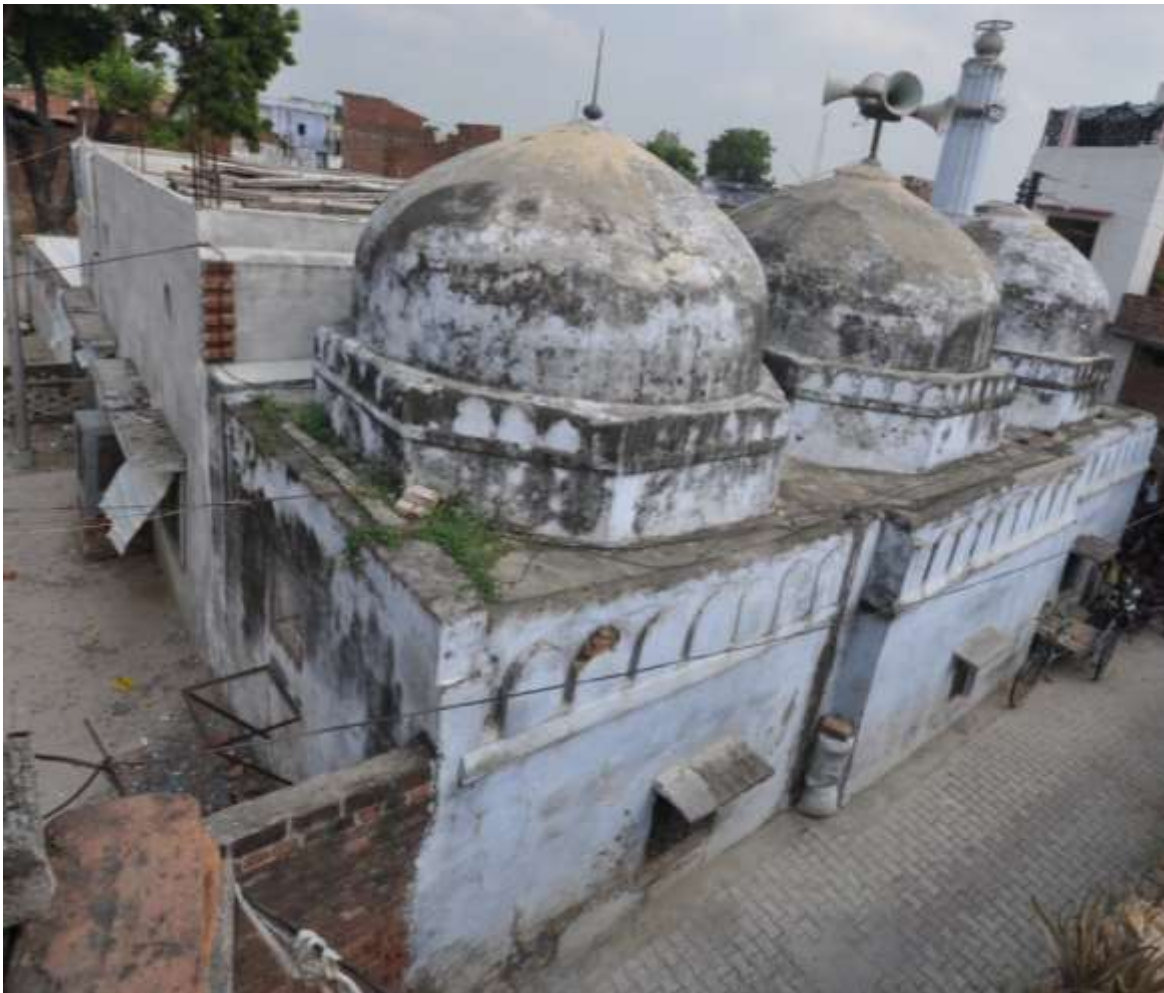
Fig. 32: Rear façade and Domes, Daire Wali Masjid
