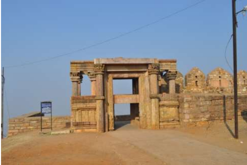
Fig. 17: Eastern façade of Parmāla gate
