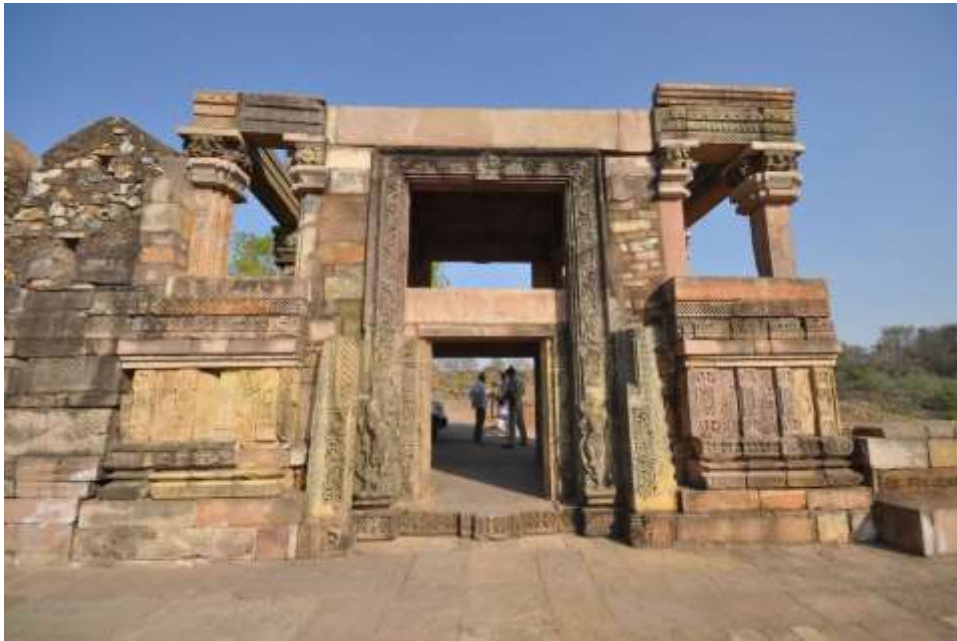
Fig- 18: Western façade of Parmāla gate
