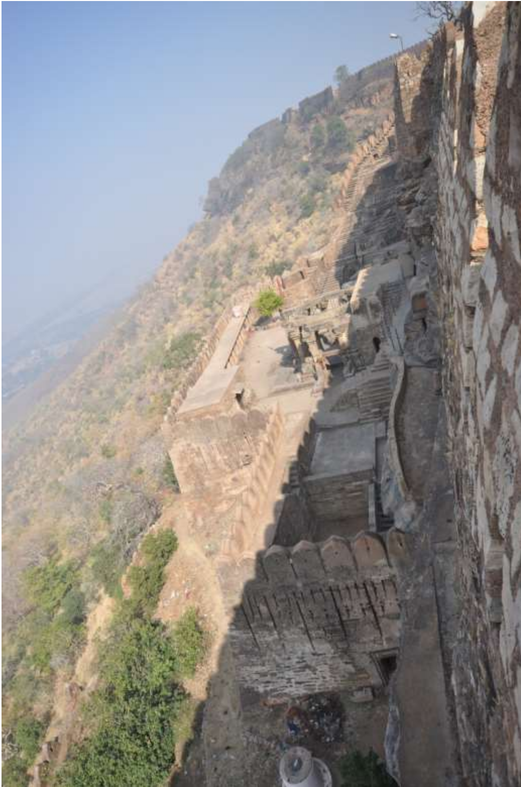
Fig. 38: General view of first enclosure of Nilkaṇṭha compound from South
