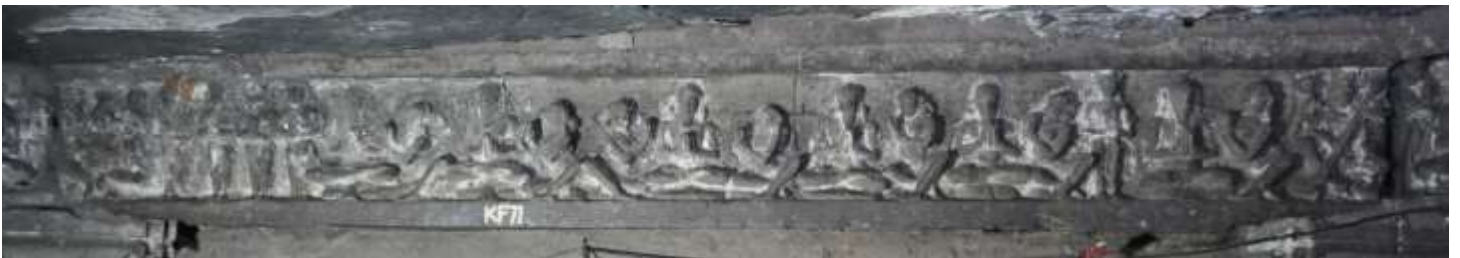
Fig- 14: Lintel of the second wall
