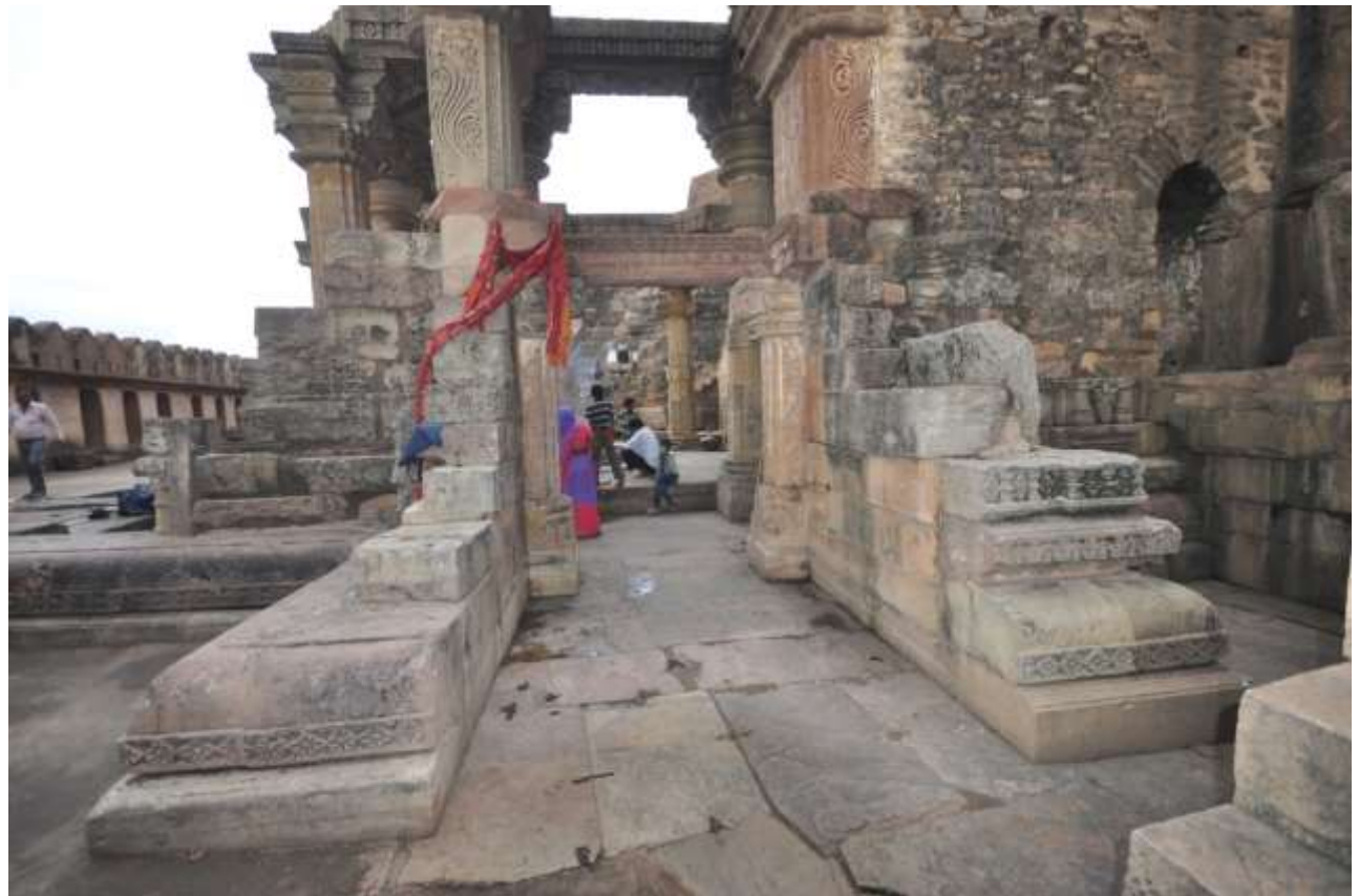
Fig. 3: View of southern entrance
