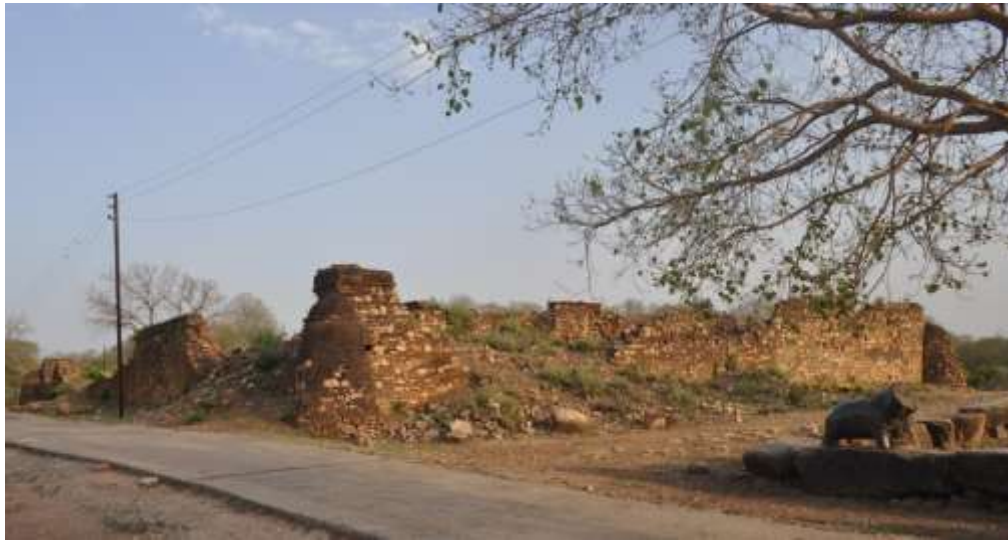
Fig. 1: View of Jauhrā from north-west
