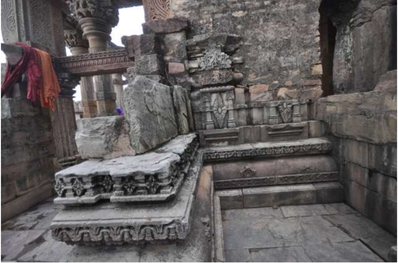
Fig. 2: The view of southern entrance
